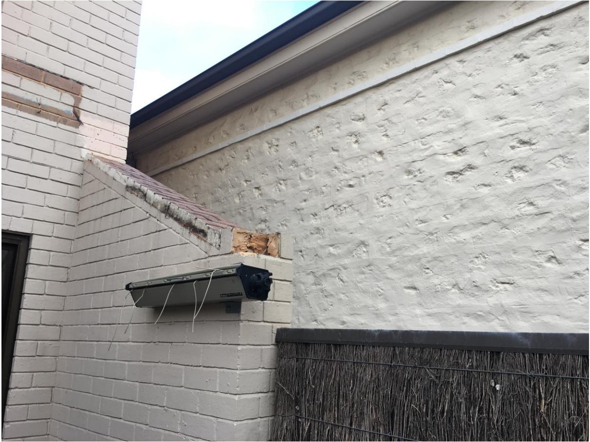
Photo 6 – View of existing boundary wall abutting the boundary with 81-85 Hill Street
