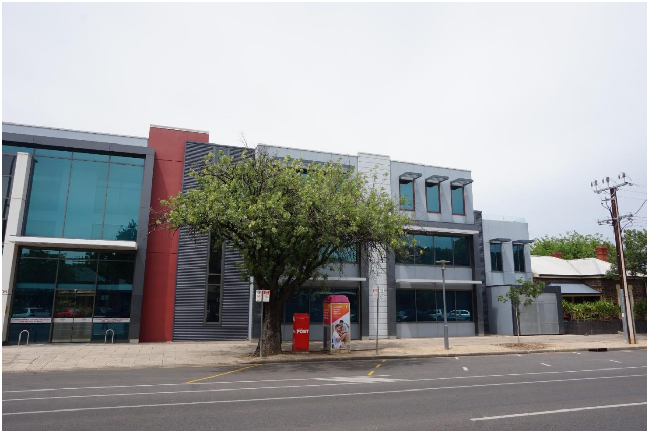
Photos 8 and 9 – Examples of more moderately scaled development in Halifax Street to the east of subject site
